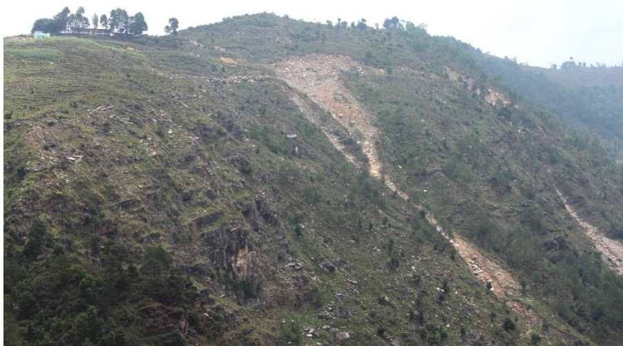
A landslide which occurred in Bhir gaun of golche in Jugal Rural Municipality. Due to this landslide, people living across Sehera river have difficulty accessing the school located beyond the landslide as the landslide damaged the path as there's no suitable bridge to cross the river
