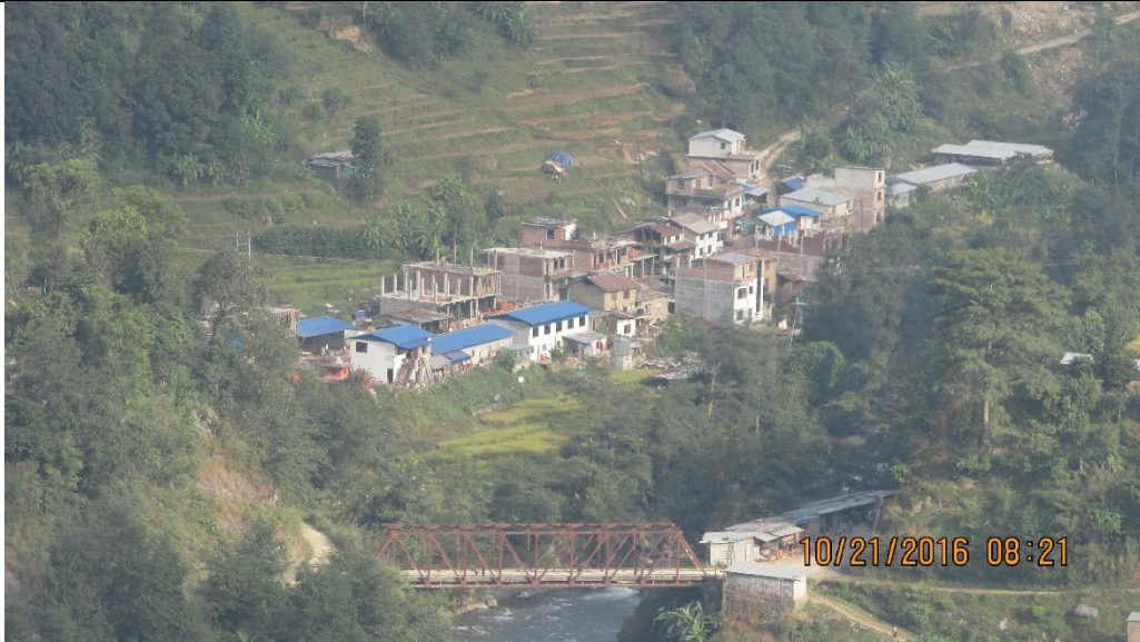
Chanaute Bazar and bridge in Helambu during 2016
