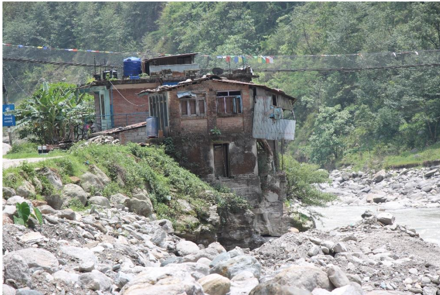
House at flood risk zone
