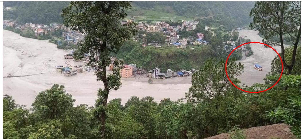
Wide view of damage of melamchi flood
