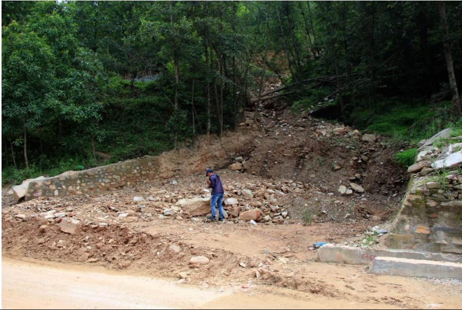
The flood of aanbu kholsa (आँबु खोल्सा) 2 years back at Balephi Rural Municipality caused the damage to two houses destroying the agricultural land as well.
