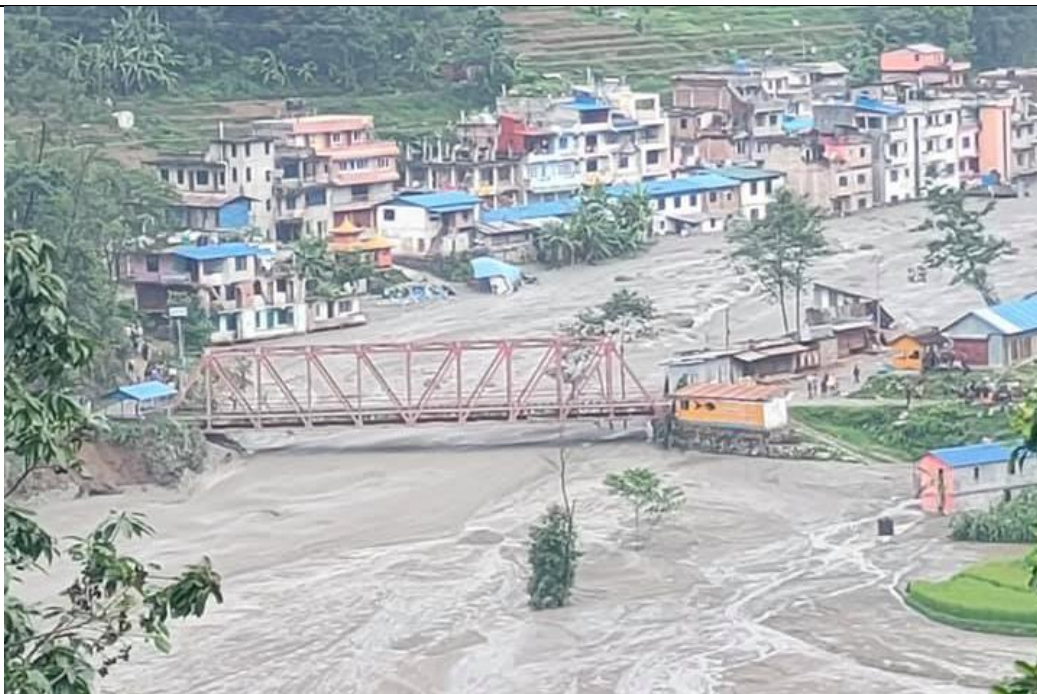
Chanaute Bridge in Helambu which was washed away in second flood August 1, 2021
