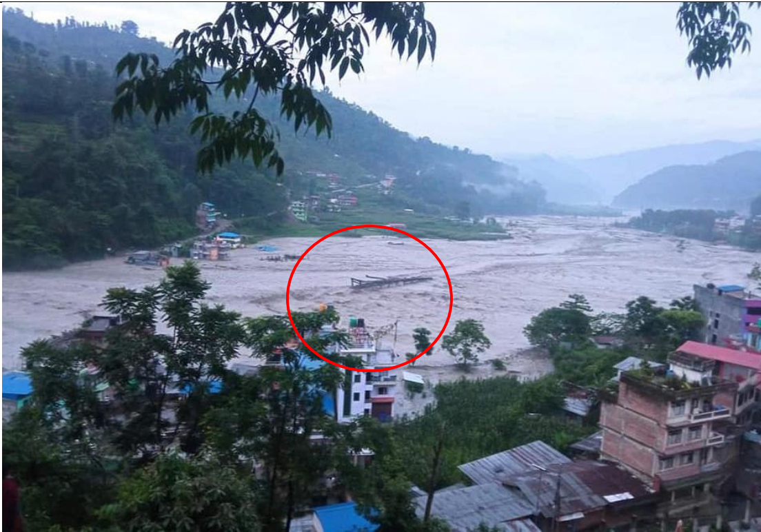
Bridge Washed away by Melamchi Flood
