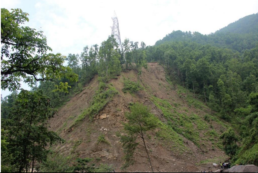
High tension line at risk of slide due to road construction on the way to Jalbire (जलबिरे) from Balephi (बलेफी) bazar of Balephi Rural Municipality
