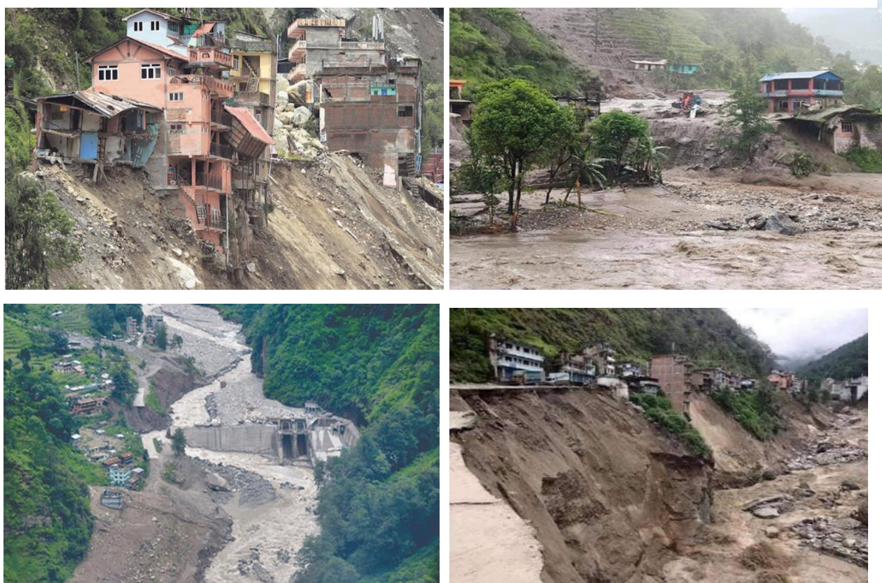
Figure 3: Damaged dam of the Upper Bhotekoshi Hydropower Project after flooding on 5 July 2016 on the Bhotekoshi River in Sindhupalchok district and flood caused in the downstream. (Sources: News Media)
