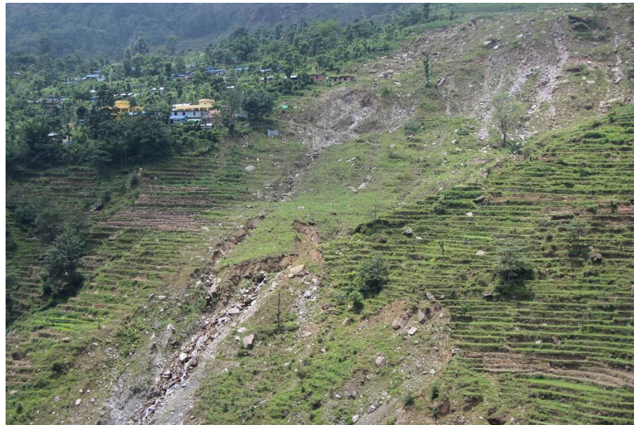
Close up view of Nakhkuche (नाखकुच्चे) landslide at ward no 7 of Barhabise Municipality with relocated settlements
